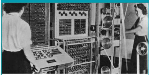
Codebreakers during World War 2 constructed the Colossus computer in 1943. This enormous machine was the world's first electronic, programmable computer.
